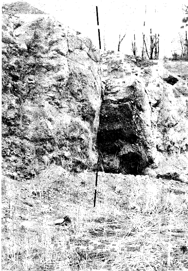
A. Shear fault cutting coarse red arkose of the Middleton basin. Shallow, horizontal grooving of fault surface not visible on photo. Triassic border-fault crosses quarry bench obliquely in foreground.
